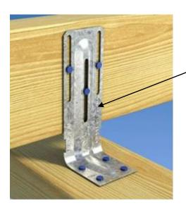
Traditional and compliant method of restraining tops of internal partitions.
